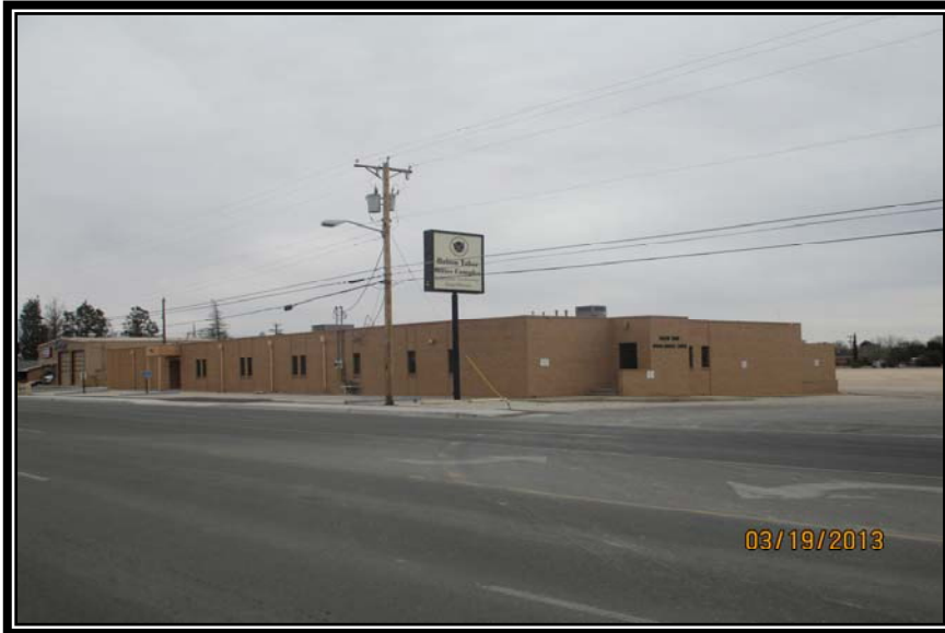
LOOKING SOUTHEAST ACROSS EAST BENDER BOULEVARD AT SUBJECT
