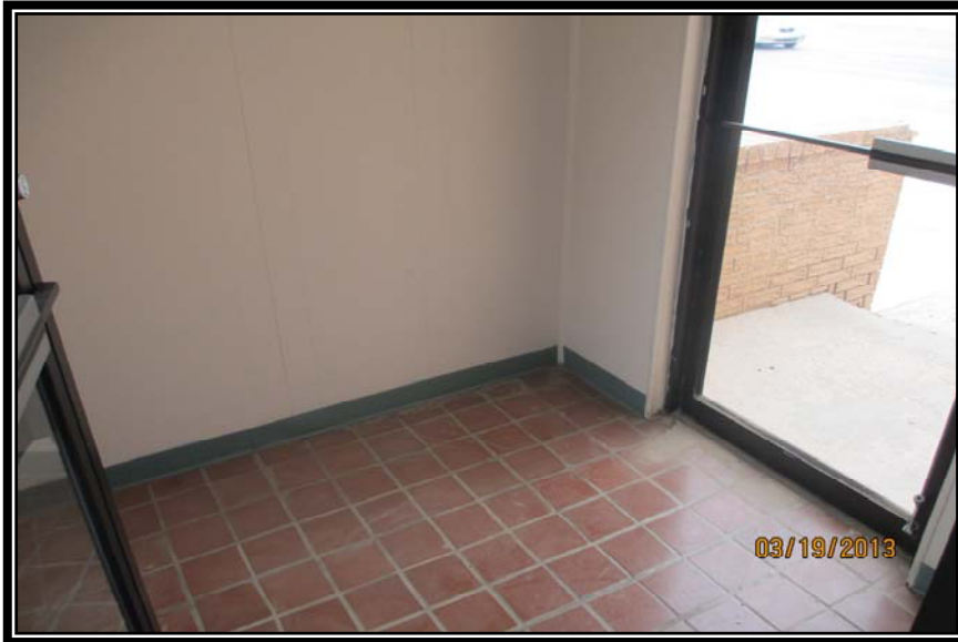
WEST END ENTRY VESTIBULE
