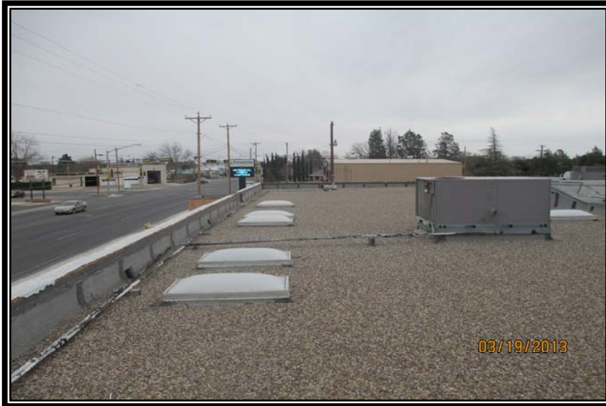
VIEW OF ROOF, HVAC UNITS, AND SKYLIGHTS LOOKING EAST
