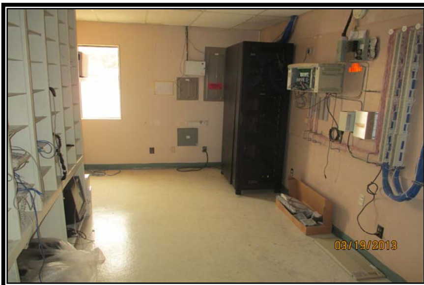
STORAGE ROOM / ELECTRICAL / TELEPHONE ROOM
