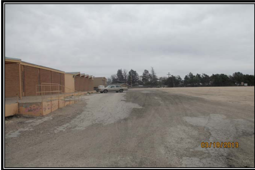
REAR (SOUTH SIDE) OF SITE – NOTE POOR CONDITION OF PAVING/STRIPING
