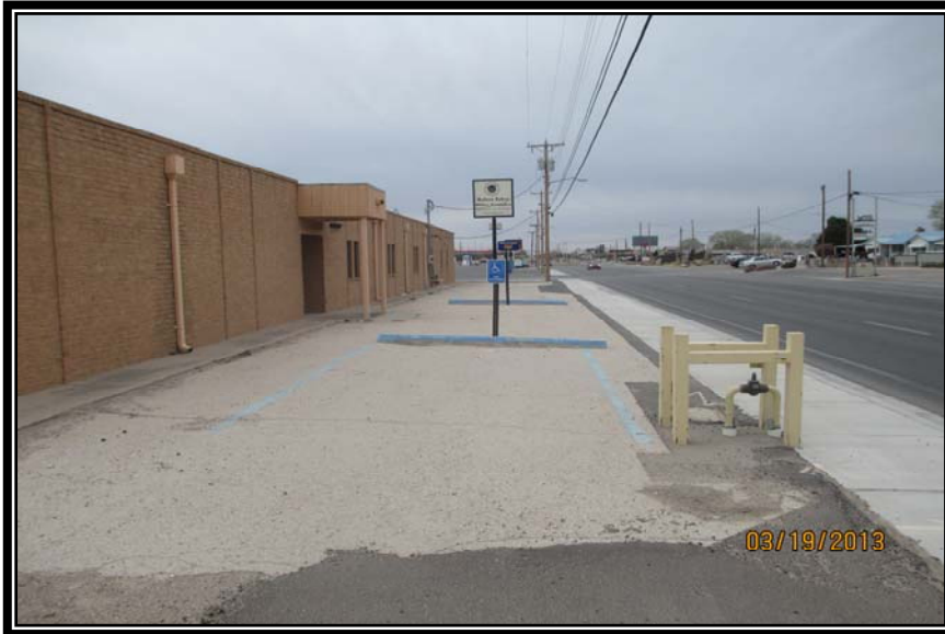
LOOKING WEST AT FRONT HANDICAP PARKING AREA
