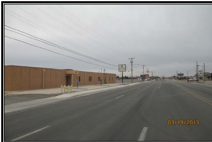
LOOKING WEST ON EAST BENDER BOULEVARD – SUBJECT ON LEFT
