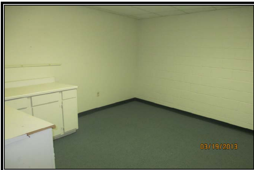
TYPICAL OFFICE – NOTE LOW QUALITY CABINERY
