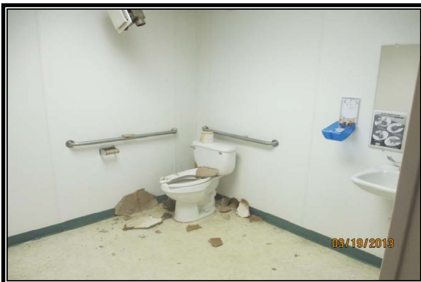
NEW HANDICAP ACCESSIBLE RESTROOM
