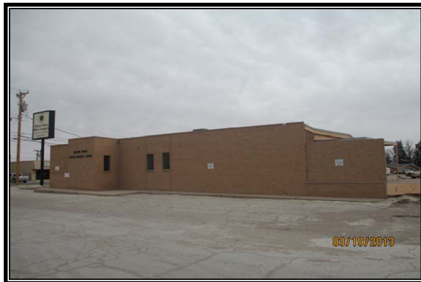
WEST END OF BUILDING
