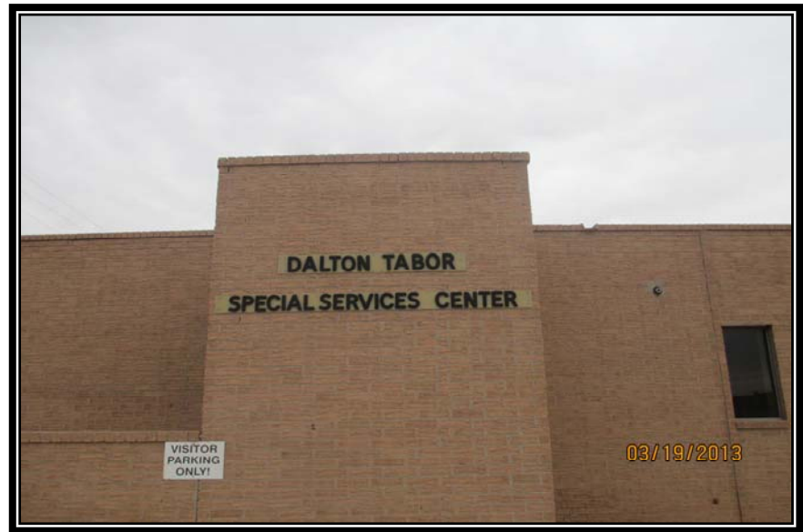
SIGNAGE ATTACHED TO WEST END OF BUILDING
