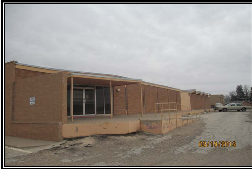
SOUTH SIDE AND LOADING DOCK ON SOUTHWEST CORNER OF BUILDING
